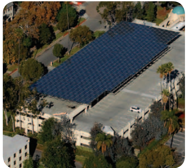
Solar now accounts for two percent of Caltech's energy portfolio, and has been deployed on 72 percent of eligible roof-top space.
