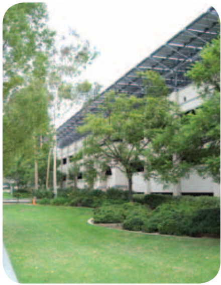
Caltech's Holliston Avenue parking structure features a 200 megawatt solar array on its roof. The installation and six others on campus have earned the institute a rebate of over $900,000 for five years of service.
