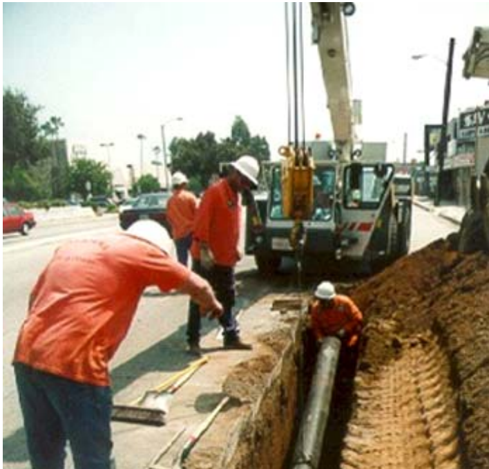
Fire Protection System Improvements
