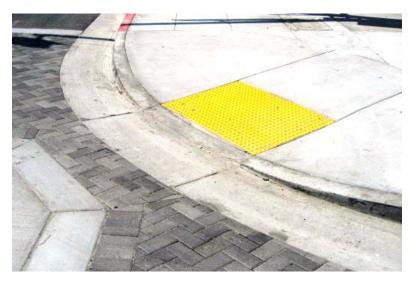
**DESCRIPTION:** This project will install curb ramps along arterial and collector streets, detectable warning surfaces on existing ramps, and tactile pedestrian push buttons at selected signalized intersections. The Accessibility and Disability Commission will work with staff to identify specific locations for these improvements.
