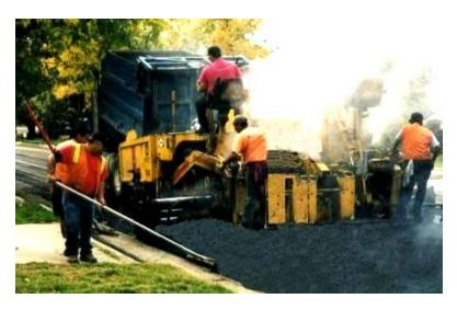
**DESCRIPTION:** This project provides for the systematic resurfacing (asphalt overlay) and slurry sealing of all asphalt streets throughout the City at prescribed intervals. These intervals vary depending on the age of the street and traffic volume. This project also includes funds for a separate project to repair damaged concrete adjacent to the street to provide proper drainage and better ride quality.
