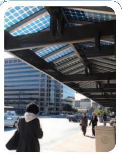
The building-integrated solar panels at the Lake Avenue Metro Station are a first for Pasadena, providing light-filled shelter as bus stop canopies, in addition to clean energy to the grid.
