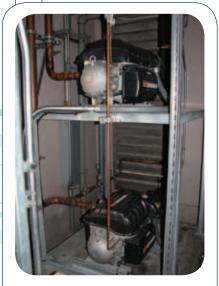
Newly-installed lightweight Turbocor compressors will help 99 S. Lake Avenue building save up to 70 percent in energy costs. PWP's Energy Efficiency Partnering Program (EEP) helped offset the cost of the upgrade.
