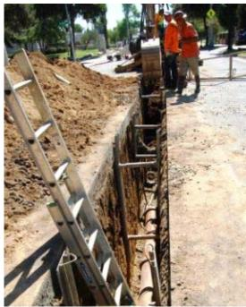
**DESCRIPTION:** This project provides for the replacement or relief of 8.5 miles of existing sewer pipes that are hydraulically deficient. This five year project will continue to address the remaining deficiencies at the following locations:
