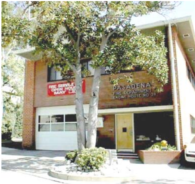
Fire Station #39 - 50 Avenue 64
