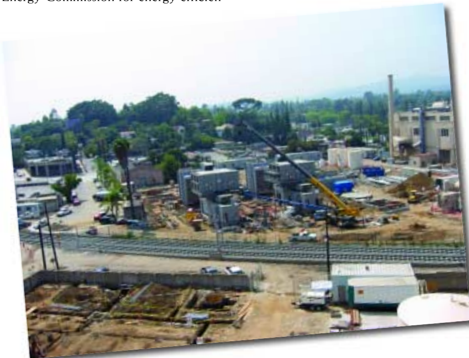
The new $82 million Glenarm Plant, shown early during the construction process.
