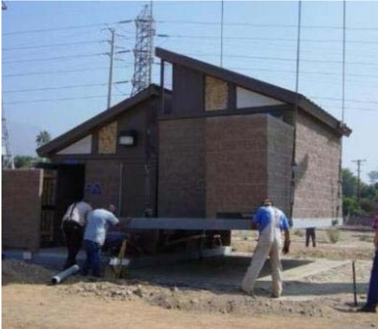
New Restroom Installation
